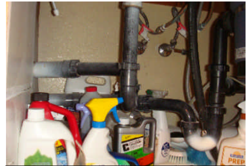
View below the sink.
