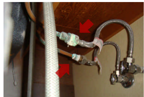
Corroded connectors.
