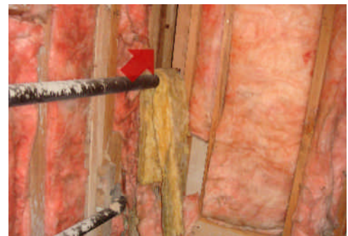
Secure insulation & install between frame.
